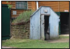
An Anderson Shelter was made to provide shelter for up to six people during an enemy air raid. Courtesy: Matinvl via Wikipedia
